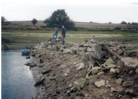
The dam at Derby Hills, photographed on one of its rare emergences from under the water
