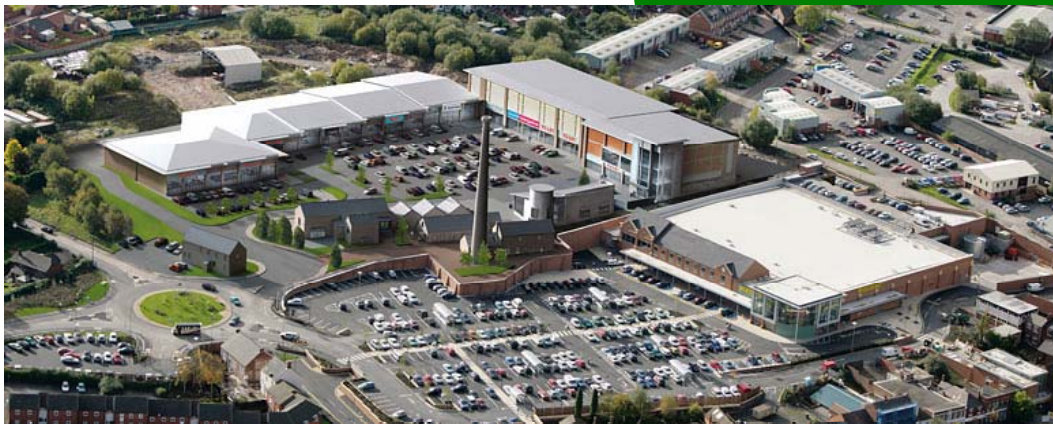
New mixed-use residential, retail and leisure scheme under construction in Swadlincote town centre
