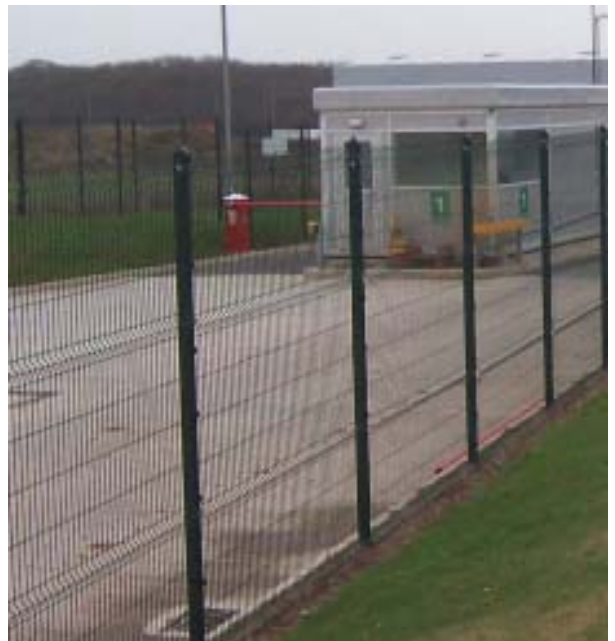
Fig.4. Weld mesh fence, Dove Valley Business Park
